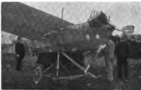
THE DAMAGE DONE TO AN ANTOINETTE BY A HEAVY "HEAD-ON" LANDING
